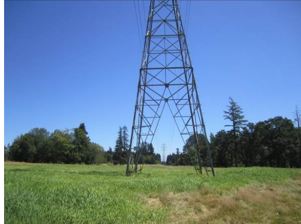
Typical view powerlines (to the south)
