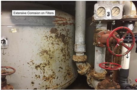
Extensive Corrosion on Valves Metal Piping in Pool System
