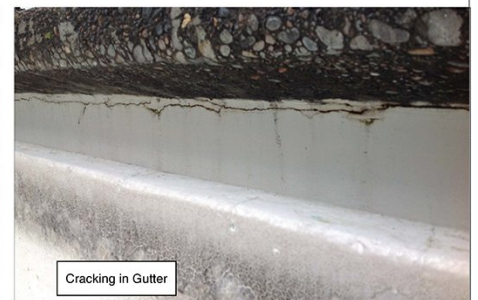
Insufficient Gutter Drop-Out
