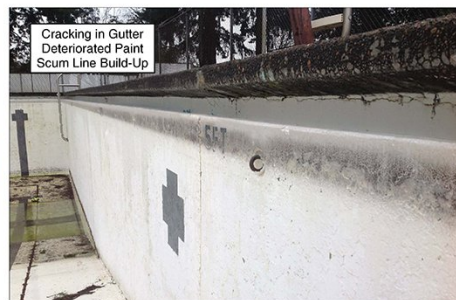
Cracking in Gutter
