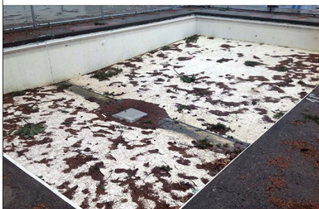
Deteriorating Pool Paint
