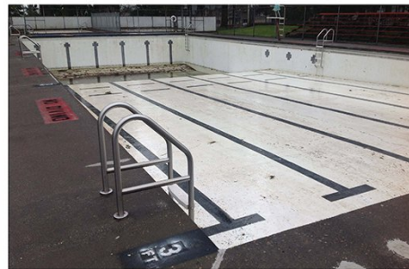
Cracking in Gutter Deteriorated Paint Scum Line Build-Up
