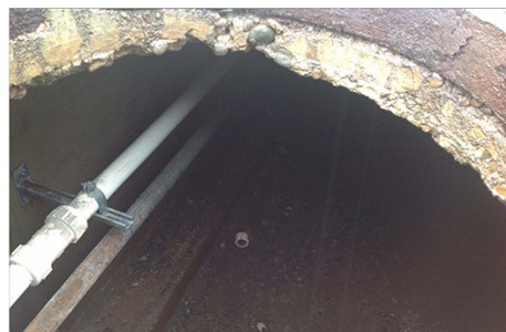
Cracking in Gutter Deteriorated Paint Scum Line Build-Up
