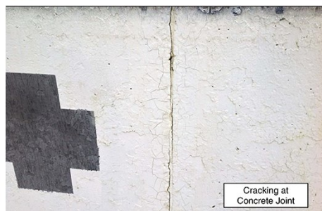
Deteriorating Pool Paint
