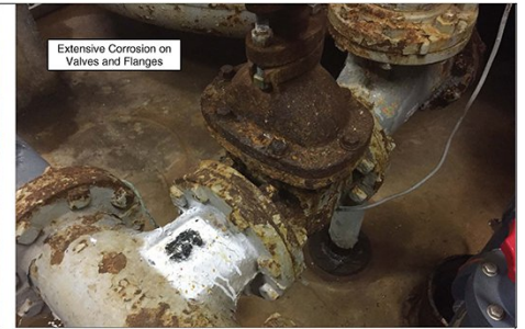
Paint Chipping, Peeling, and Flaking Away
