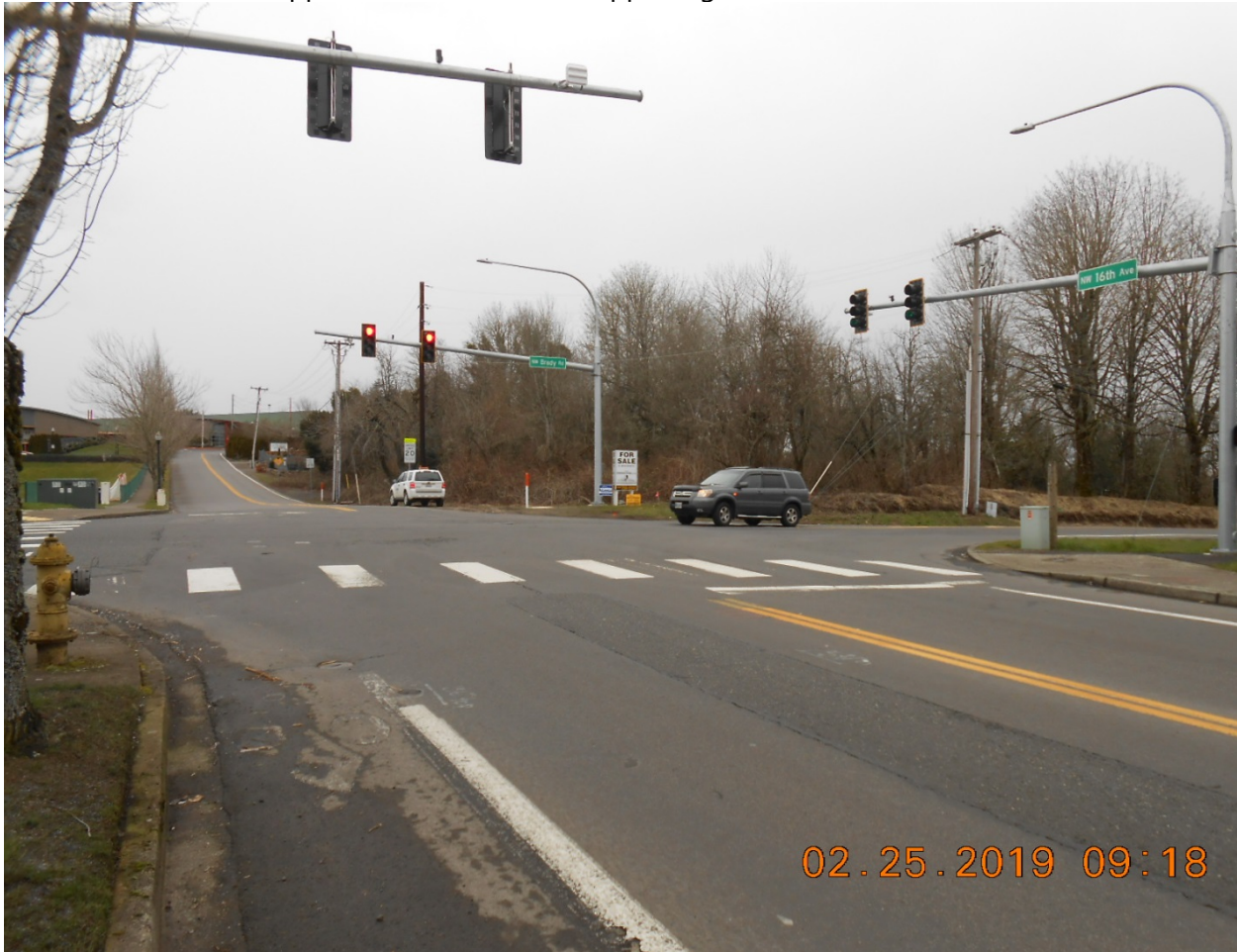
Camas School District Traffic Signal Improvements at Intersection of NW Brady Road & NW 16 th Ave. (looking west)
