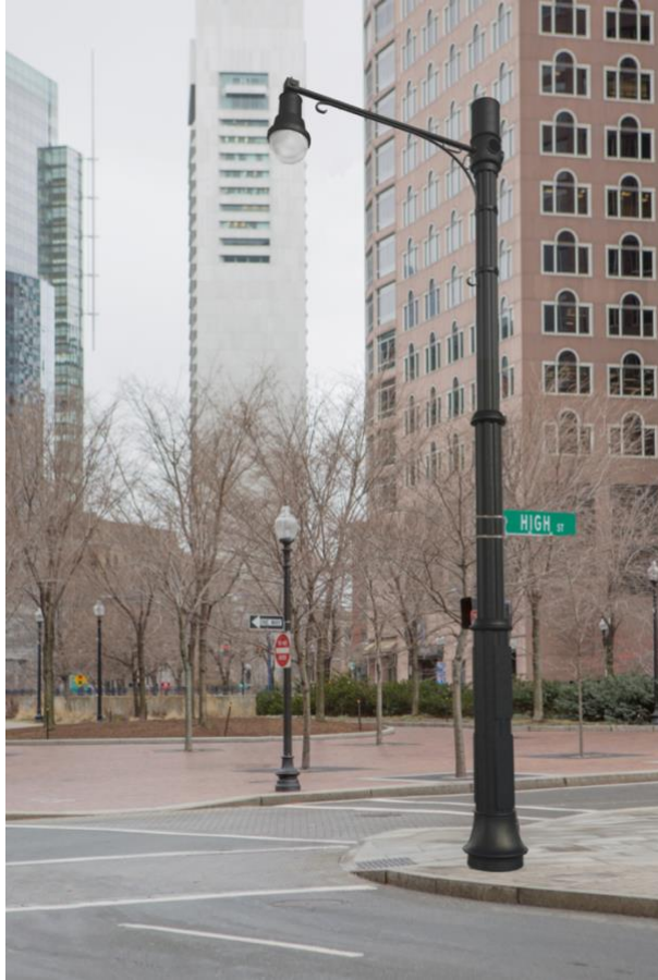
Example of a new small wireless facility pole that is compatible with the streetscape, likely better than attempted collocation on shorter acorn light poles in the background
