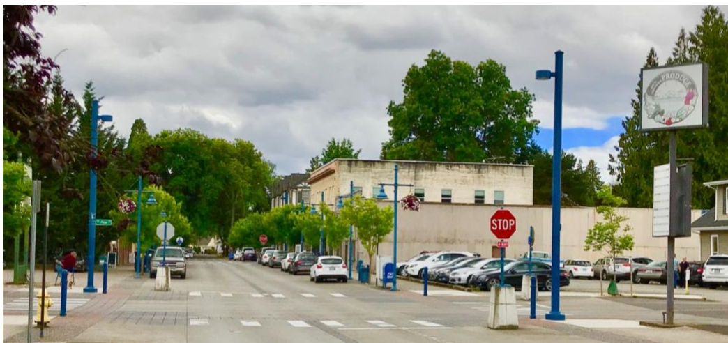
Downtown with Different Pole Types – larger intersection poles are likely better opportunities for small wireless facility collocation than pedestrian streetlight poles
